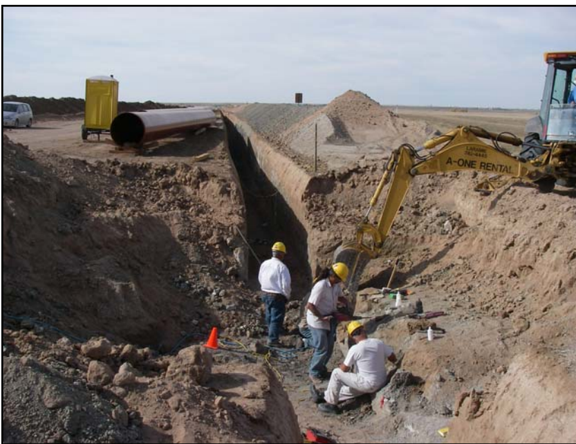
Figure 1: Excavation of the Laramie Pipeline Dinosaur.
