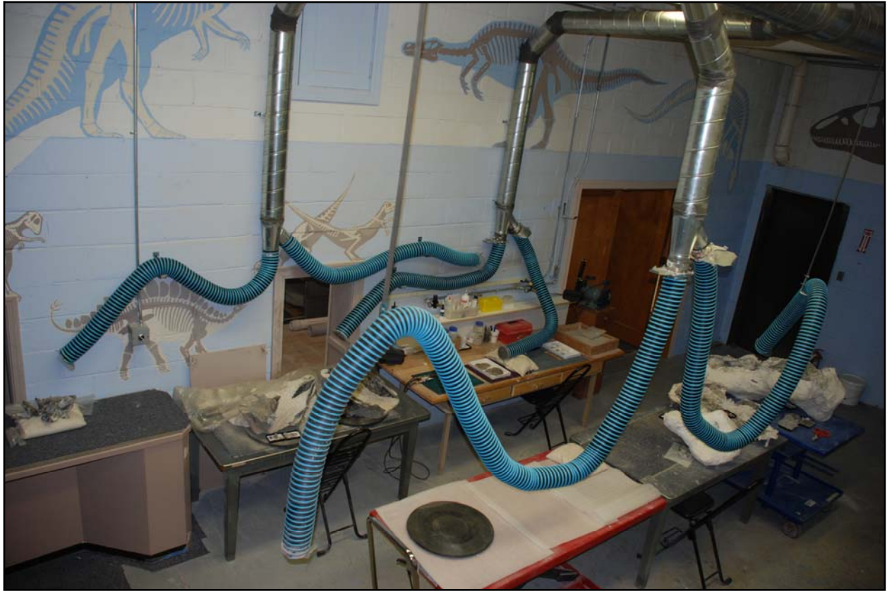
Figure 1 (above). New duct work at UFH
